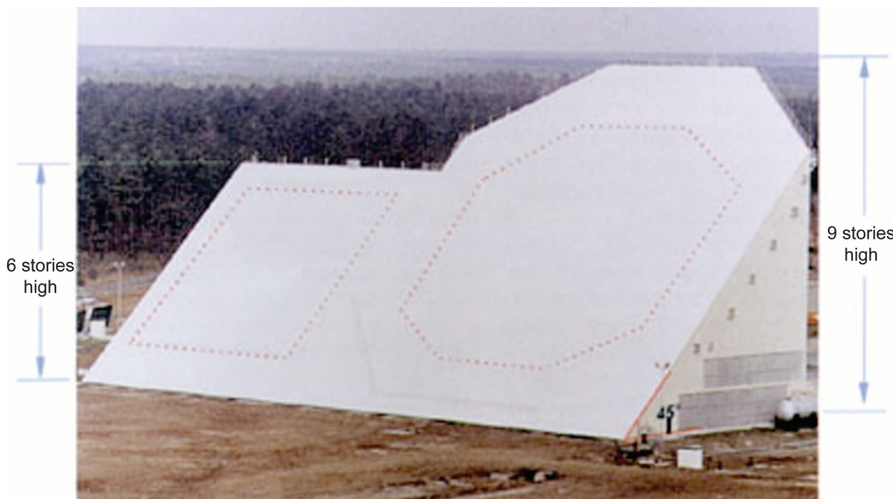
FIGURE 6. Photograph of the phased array radar AN/FPS-85 at Eglin Air Force Base in Florida, U.S.A. The transmitter is the smaller six-story-high structure on the left that supports 5134 transmitting units. The nine-story unit on the right supports 4660 receiving units. Photo taken April 6, 2011, by the author during an authorized visit to the installation.
