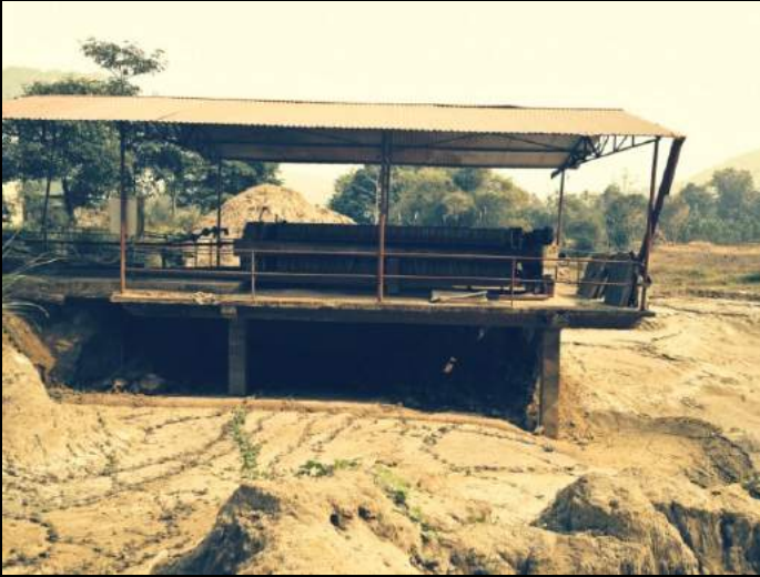
Final Filtration System – Pond Missing
