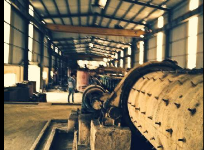
Primary Crusher, Flotation Cells and Primary Filters
