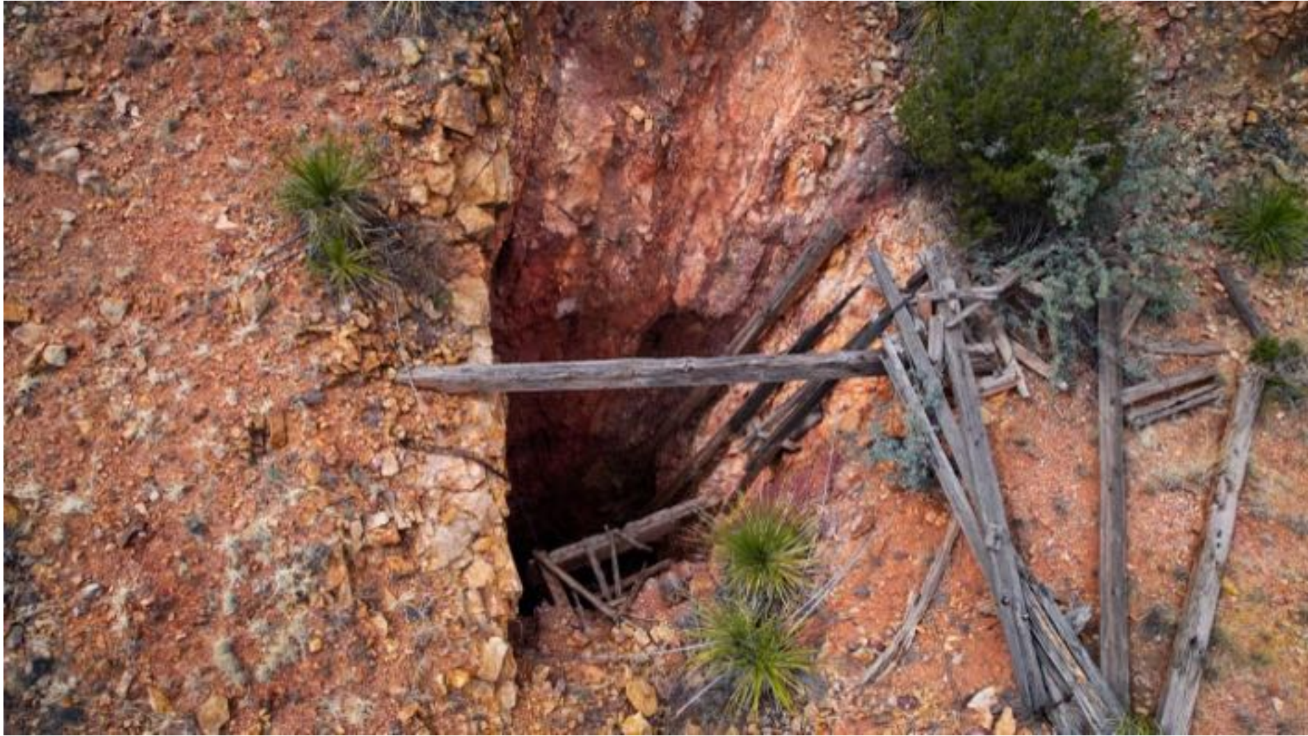
Figure 2.18 – Overhead view of the main vertical shaft (200') in the Northern Ore Body.
