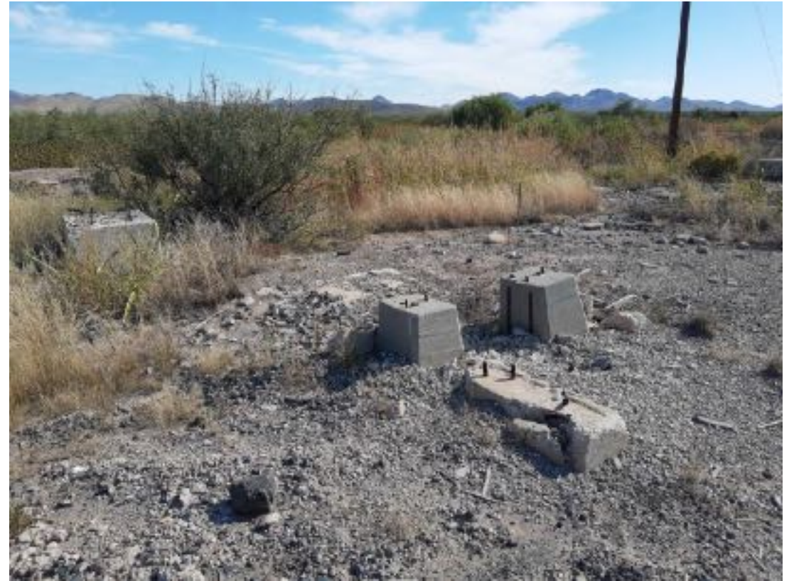
Figures 2.11a and 2.11b – Concrete structures used to support pumps at old Hot Wells station, hotel, and bath house. Photos by BK Darling.
