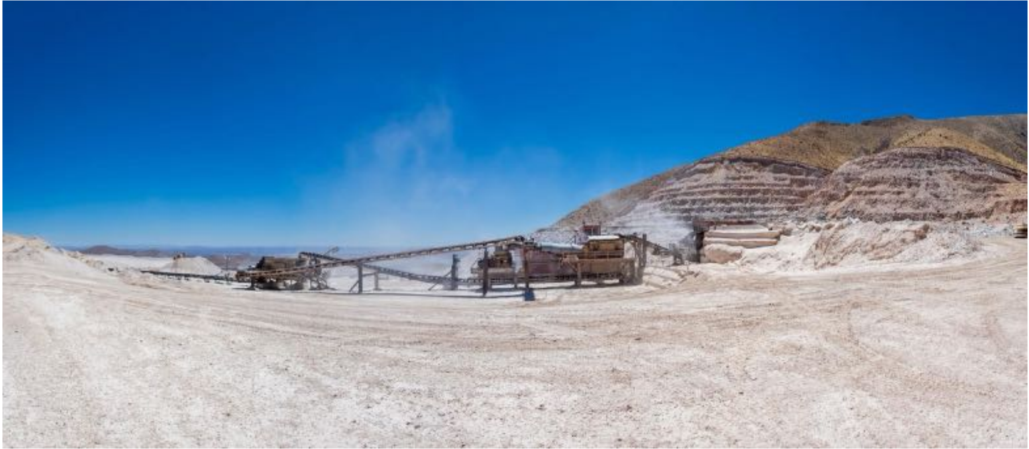
Figure 1.07 - Wide-angle view of rock crusher and main quarry. Benches cut to stabilize slope and to allow for further development of the quarry are seen above quarry wall in background. Photo by Paul Warren
