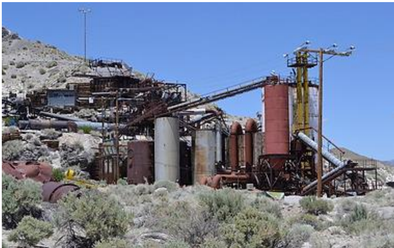
Figure 8. American Perlite Plant. From American Perlite.com. Accessed Feb. 20, 2023.
